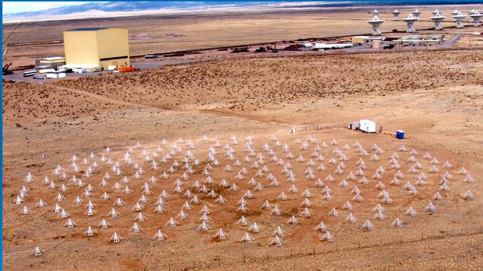
LWA-1 New Mexico near the VLA 256 antenna elements
