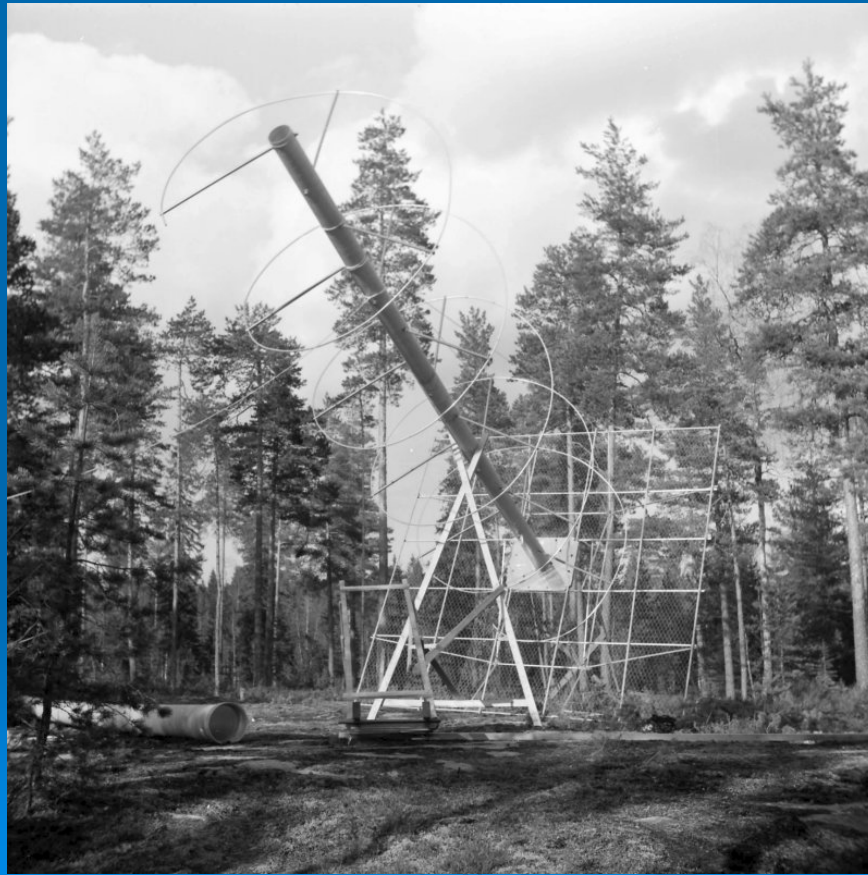
A huge right hand circular helix – likely erected by Riihimaa in Finland
